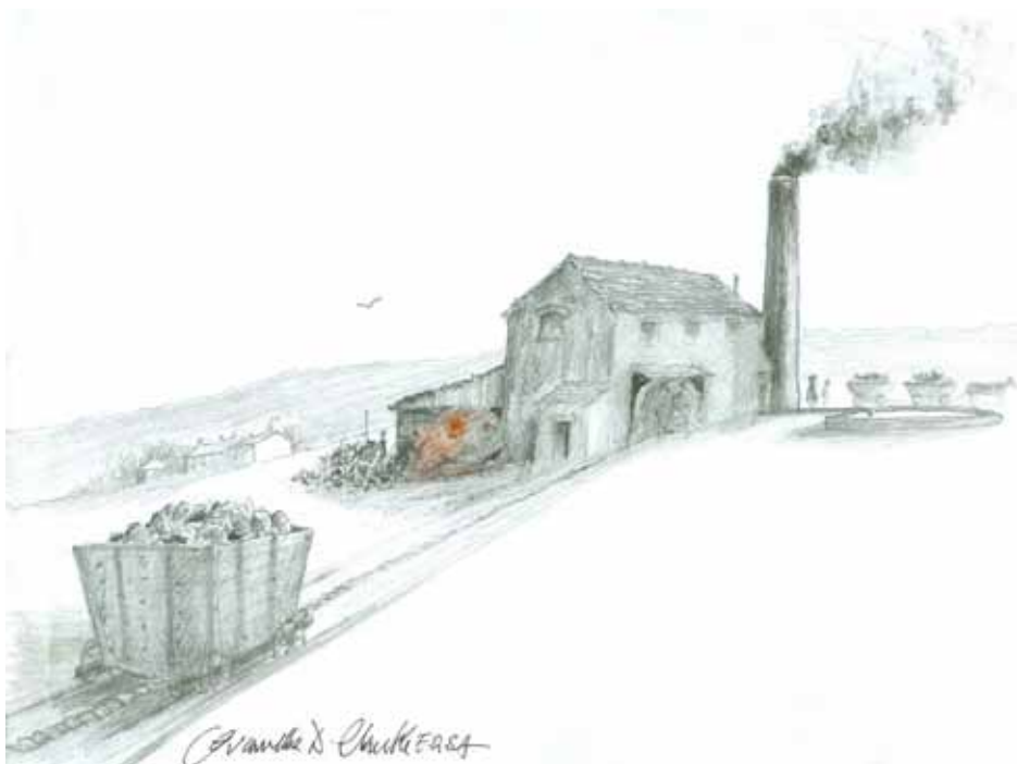
Coal waggon being hauled up the inclined plane towards the Black Horse engine and boiler house Original sketch © Granville Daniel Clarke 2014
