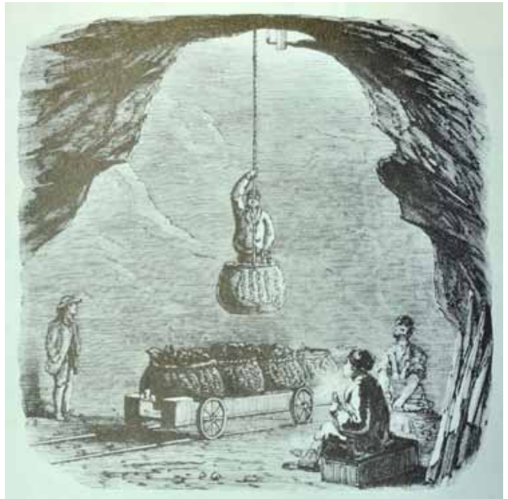
Corves of coal being raised from pit bottom From the Royal Commission Report on the employment and conditions of children in mines and manufactories (1842)
