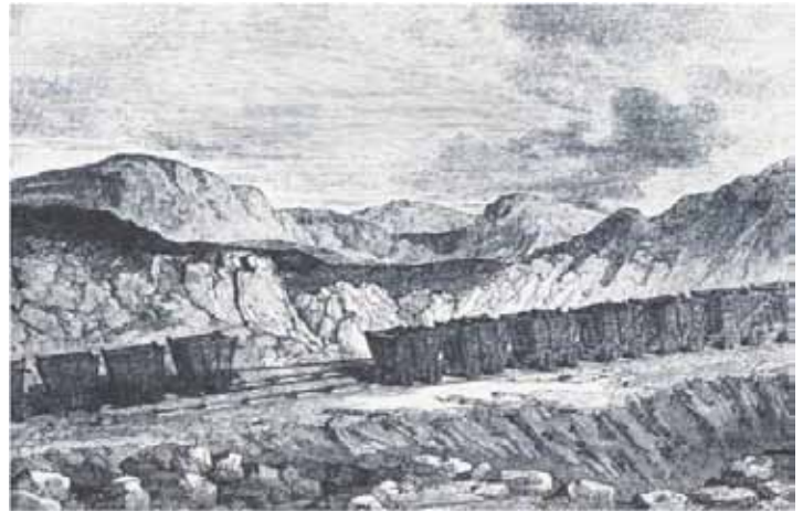
Waggons on an inclined plane Reproduced by kind permission of Barnsley Archives and Local Studies
